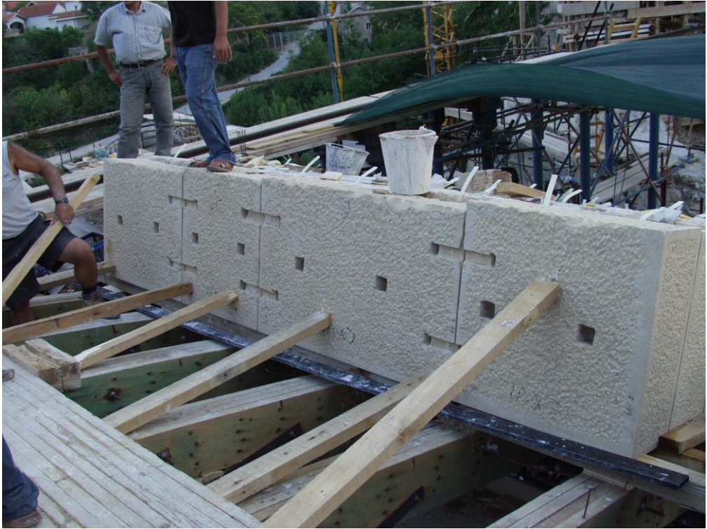
Picture 15: The last rows of stone arch
