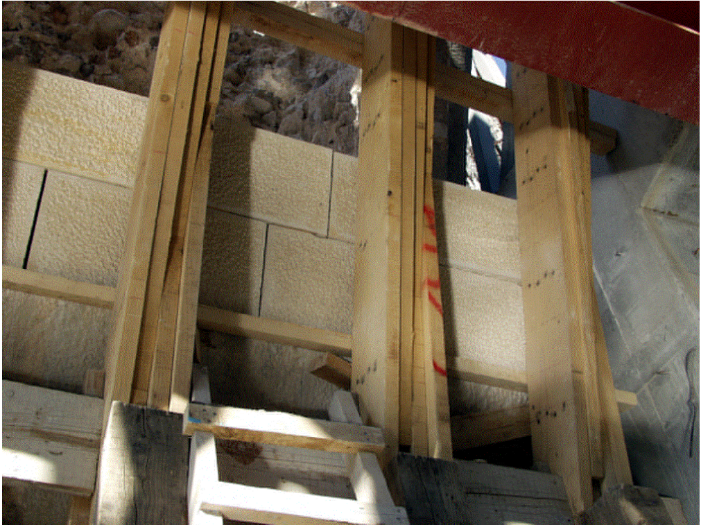
Picture 14: The first rows of stone arch
